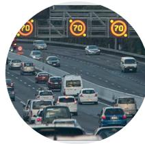
Safety and network management is improved with an upgraded motorway alignment and through technologies such as variable speed limits, ramp signalling, and incident and congestion detection capability.
